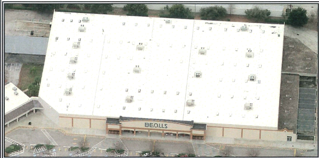
(A) PARTIAL NORTH ELEVATION - EXISTING CONDITION
